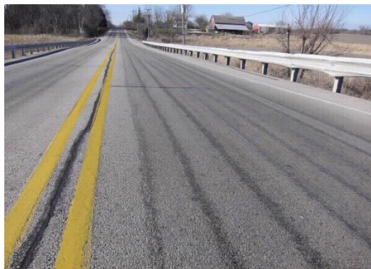
Striping on roadway from application of liquid brine
